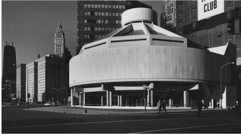
Seventeenth Church of Christ, Scientist, Chicago Designed by Harry Weese and Associates, 1968 Photo by Orlando Cabanban Printed with permission from W.W. Norton & Company
